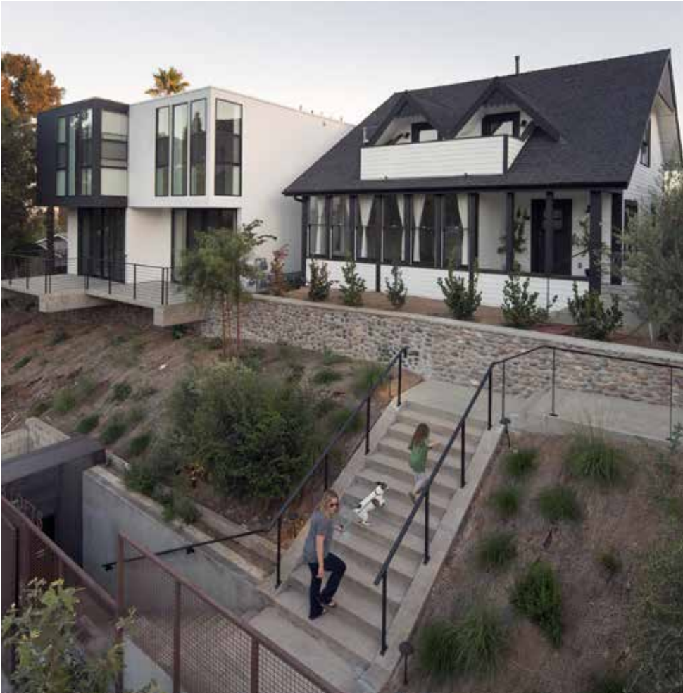
The house, east building, and front yard, viewed from Broadway. At left, the east building's foundation cantilevers out over the hillside and a historic cobblestone retaining wall.
